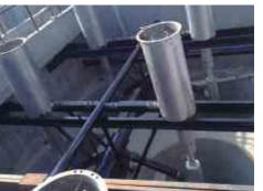
MG-CSF continuous sand filter is developed and improved upon traditional sand filter, which has been used in the Europe, the United States and other advanced countries for many years. Besides sand and air, it doesn't need any power equipment or valves. Therefore, the input of labor and material can be reduced a lot. Moreover, the equipment is easy in operation and can save man power and source. Its characteristics are as follows:
